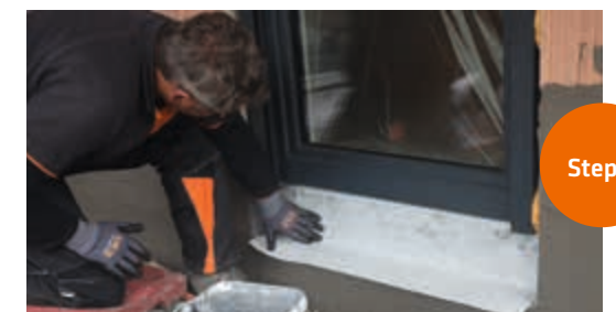
Lay the PCI Barraseal Ready Vlies fabric over the entire surface of the fresh layer of PCI Barraseal Ready and press down carefully*
