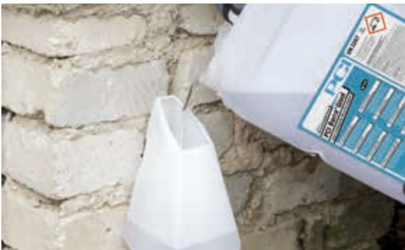
Application of a damp course to provide protection against rising damp using PCI Barra Gisol
