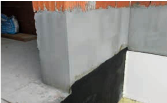
Intermediate waterproofing layer with PCI Barraseal
