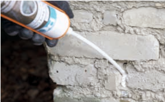
Injection of a horizontal damp course using PCI Barra Creme
