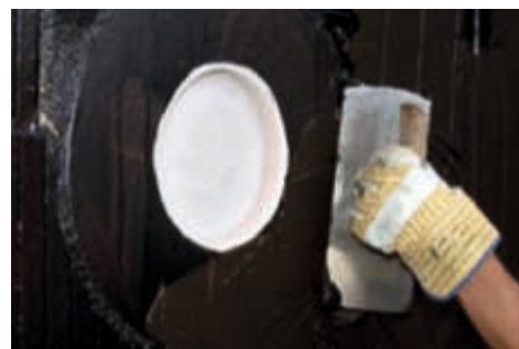
Installation of PCI Pecimor 2K on a flange
