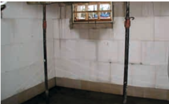
Moist masonry in a cellar
