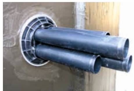
Transition to a multiple-service entry point waterproofed using PCI Barraseal Turbo or PCI Barraseal Turbo 1K
