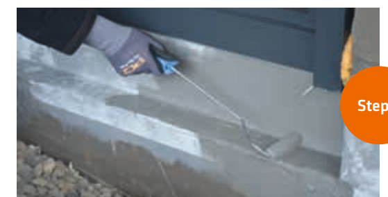
Apply a second layer of PCI Barraseal Ready wet on wet over the entire surface of the PCI Barraseal Ready Vlies fabric
