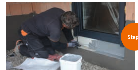
Apply PCI Barraseal Ready to the prepared substrate with a short-pile roller or brush
