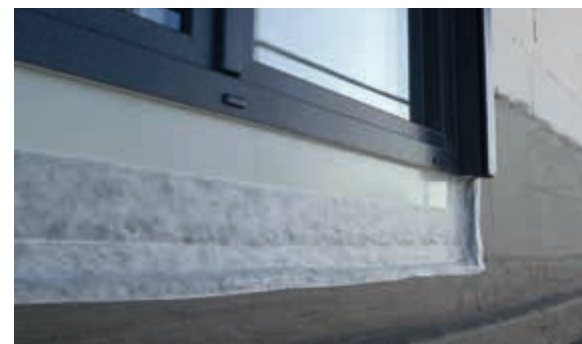
Connection to window element using PCI Pecithene Fix fixing tape
