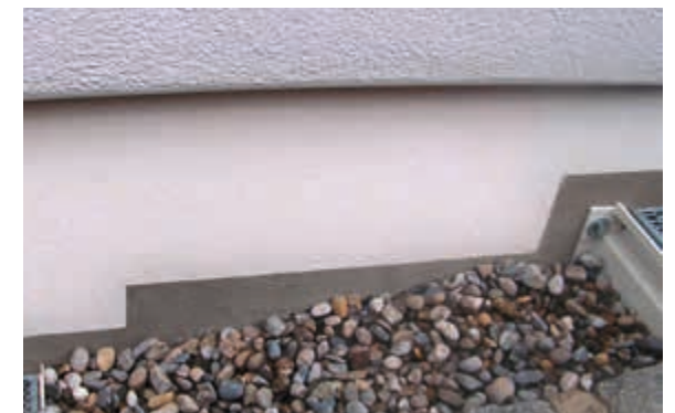
Waterproofing applied using PCI Barraseal Turbo or PCI Barraseal Turbo 1K around ground level may be left exposed, painted over or covered with render
