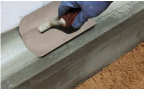
Installation of a waterproof concave molding with PCI Polyfix plus L
