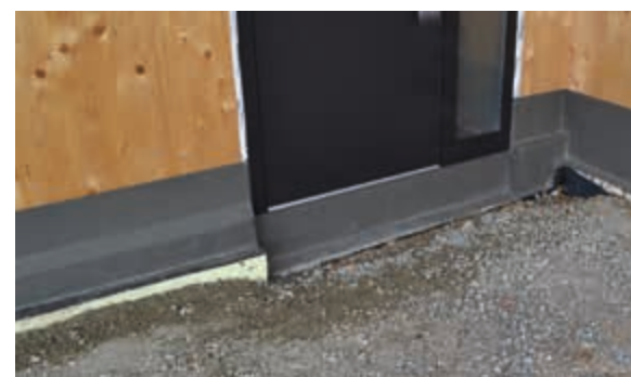
Transitions between PCI Barraseal Turbo or PCI Barraseal Turbo 1K, waterproofing tape and window element
