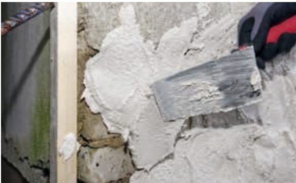
Application of PCI Saniment 2 in 1 as a combined repair mortar and fairing coat
