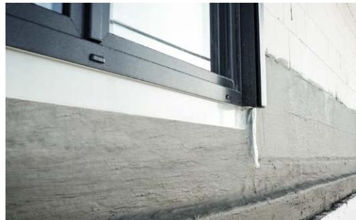
Reliable waterproofing of full-length windows, transitions or complex geometric shapes.
