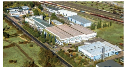
Plant in Lutherstadt Wittenberg
