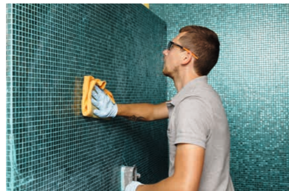
Very easy grouting without any residual slurry with PCI Durapox Premium Multicolor.
