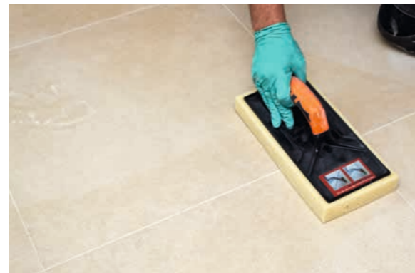
The very fine mortar structure and the strong flank bonding are special features of PCI Nanofug Premium, even in very narrow joints.
