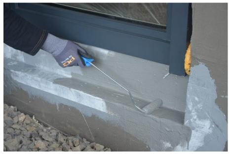
PCI Barraseal Ready in the system with PCI Barraseal Ready Vlies fabric ensures maximum crack bridging properties (<u>Link</u> to high-resolution photo)
