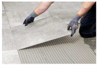
The new PCI Nanorapid fast-setting adhesive speeds up work processes and increases application convenience (<u>Link</u> to high-resolution photo)
