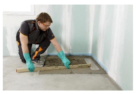
PCI Novoment Light is easy to use: effortless application and compaction with a long working time and a short drying time for rapid construction progress.
