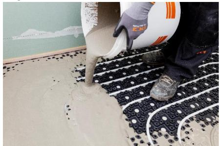
The efficient and sustainable PCI system solutions for the simple energetic refurbishment of underfloor heating systems (the picture shows the installation of a thin-film hot water heating system) (<u>Link</u> to high-resolution photo)
