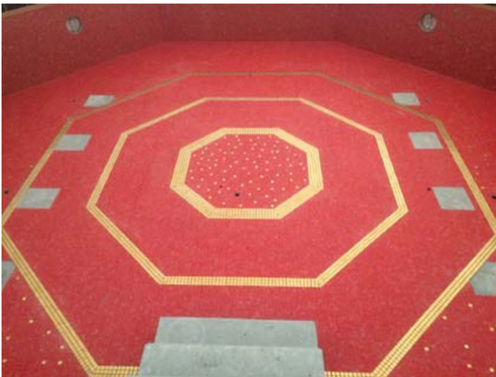
Fig. 7 and 8: The mosaic-lined pools of Kristall-Therme trimini create an exclusive and elegant impression. To ensure durable waterproofing, PCI Seccoral 2K Rapid fast-setting special waterproofing slurry was used.
