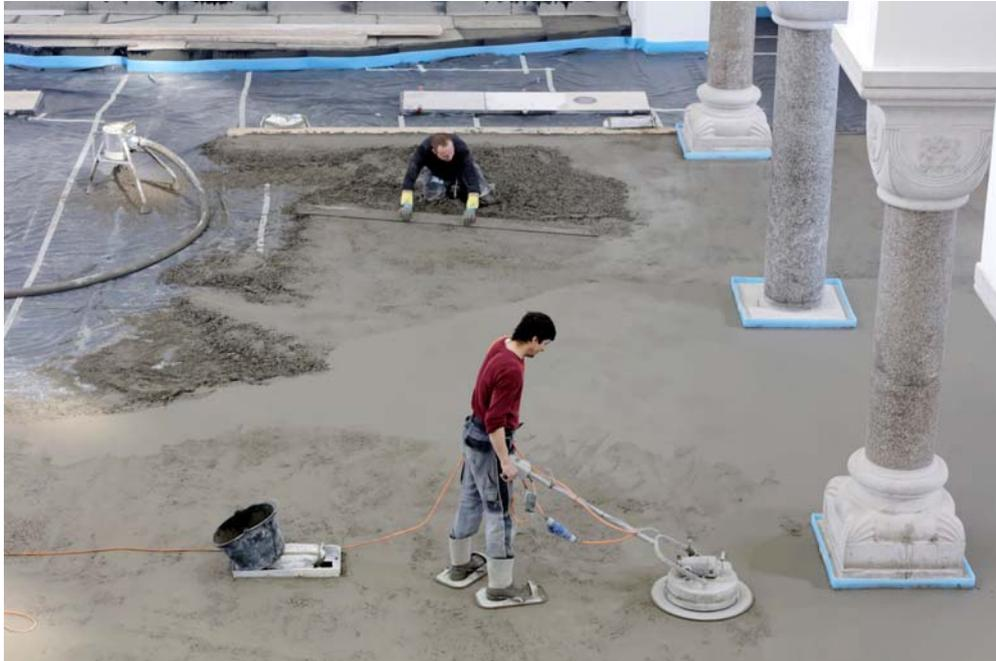
Fig. 6: The craftsmen worked hand-in-hand: following the installation and distribution of the screed material on the substrate, it was smoothed using machines.
