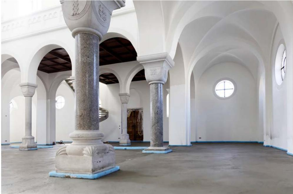
Fig. 7: The new screed in the church of St. Margaretha, with only two joints: the screed could be walked on after only one day and it was possible to lay the covering after three days.
