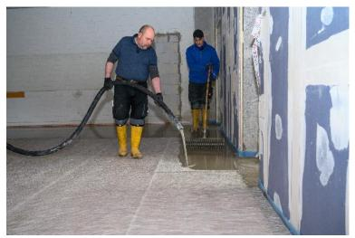
After priming with PCI Gisogrund 404, the craftsmen laid out the glass fiber reinforcement PCI Armiermatte GFM and spread the special leveler PCI Periplan Extra on top. (Link to the high-resolution <u>Photo</u>)
