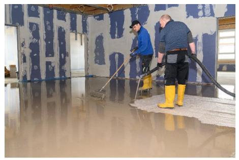
Reliable floor structure: glass fiber reinforced bonded floor leveling with PCI Amiermatte GFM and PCI Periplan Extra (link to the high-resolution <u>Photo</u>)
