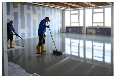
Easy processing, fast construction progress: PCI Periplan Extra is self-leveling and can be walked on after around three hours. (Link to the high-resolution <u>Photo</u>)
