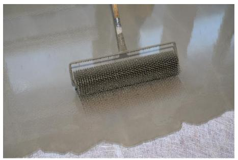
The low-dust and very low-emission floor leveler PCI Periplan Extra is suitable for layer thicknesses of 3 - 60 mm. (Link to the high-resolution <u>Photo</u>)
