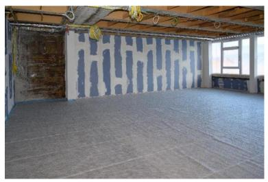
Complete refurbishment of the Löffingen secondary school: With the recommendation from PCI and the appropriate PCI products, the floor was laid on a critical substrate without dismantling the dilapidated screed. (Link to the high-resolution <u>Photo</u>)
