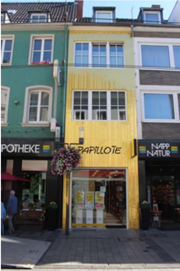
The golden facade is a real eye-catcher in the pedestrian zone of Neuss: mosaic tiles grouted with PCI Durapox® Premium. Link to high-resolution Photo
