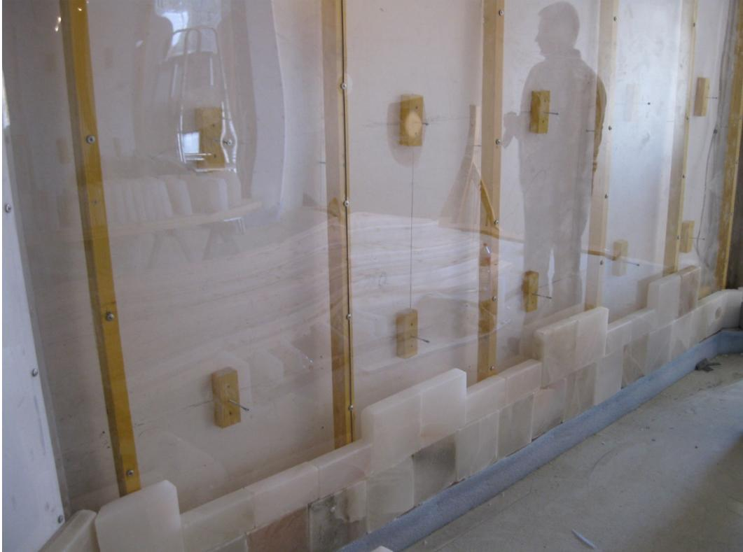
Just like the Himalaya salt, the halite salt slabs from the Salt Range in Pakistan are directly installed on the acrylic glass cladding and backlit.
