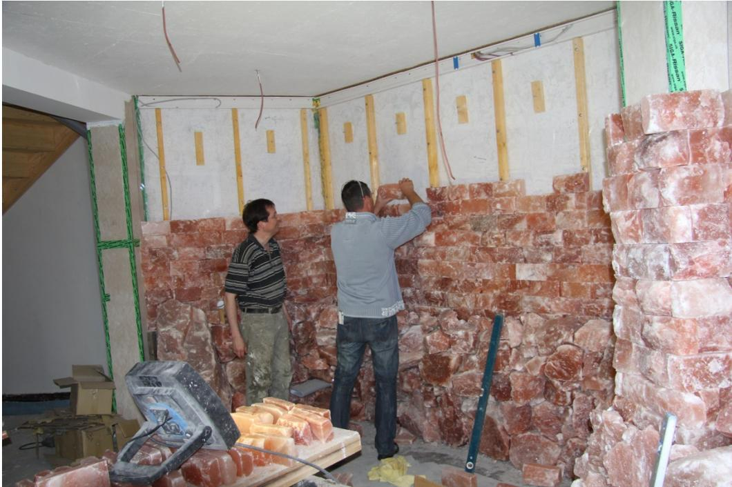
Owner and contractor at the jobsite: The salt slabs can be rapidly and easily installed with a non-sag mortar from PCI Epoxigrund Rapid, PCI Stellmittel and PCI Bauharz.
