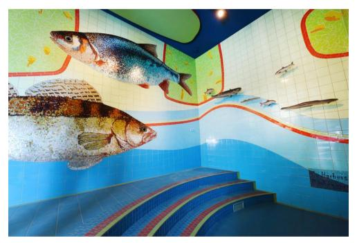
After the glass mosaic boards had been installed on site at the fish pass, the mosaics were grouted. PCI application technician Henk Nieuwenhuis provided advice and support for the project. The new epoxy resin joint grout PCI Durapox Premium was used.
