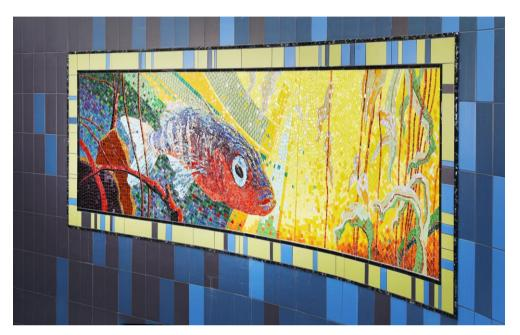
Tiler Edwin Harbers created the fish motifs with glass mosaics in about 80 different colors in his workshop. He laid the glass mosaics on Kerlite boards with PCI Nanolight White adhesive. He also used PCI products for substrate preparation.
