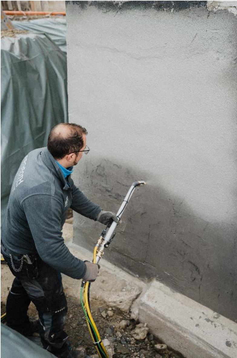
PCI Barraseal Turbo can be conveniently applied by spraying. ( Link to high-resolution photo)
