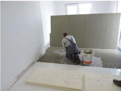
Fig. 5 and 6: To prevent voids to the greatest extent possible when laying the large fully vitrified slabs, the tilers applied the tile adhesive, PCI Flexmörtel S1 Flott, both to the prepared substrate and to the back of the slab.
