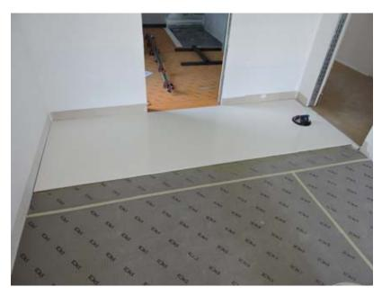
Fig. 7: To absorb stresses, the tilers installed PCI Pecilastic E insulating membrane with PCI Flexmörtel S1 Flott flexible adhesive under the tiling. The insulating and waterproofing membrane PCI Pecilastic U was used in the bathroom.
