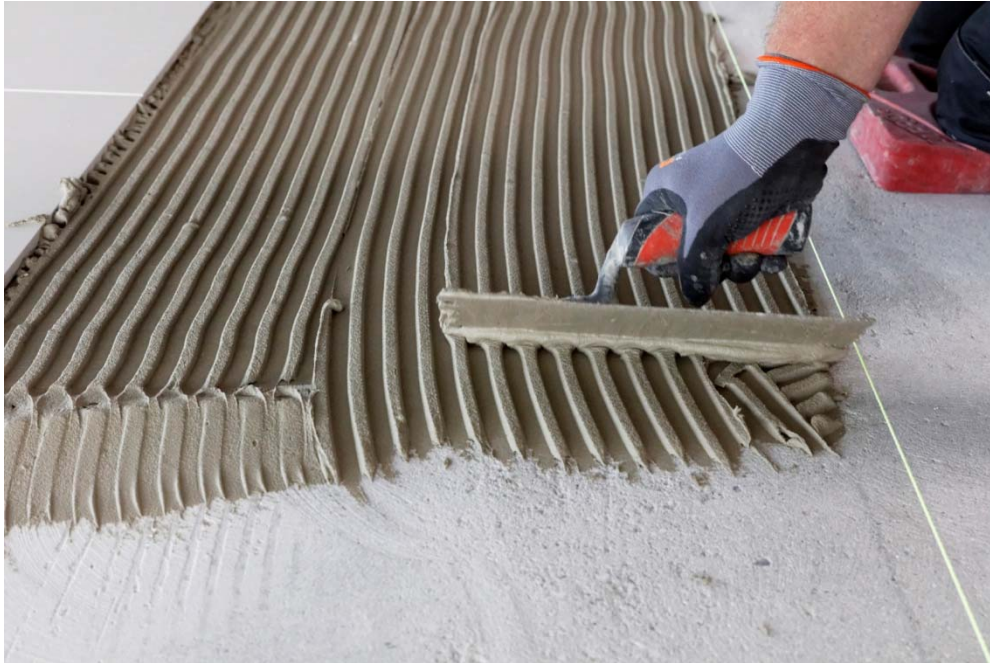
Fig. 3: The tilers apply PCI Flexmörtel S2 to the primed substrate using a notched trowel. Important: only apply as much mortar as can be covered with tiles within the specified working time.
