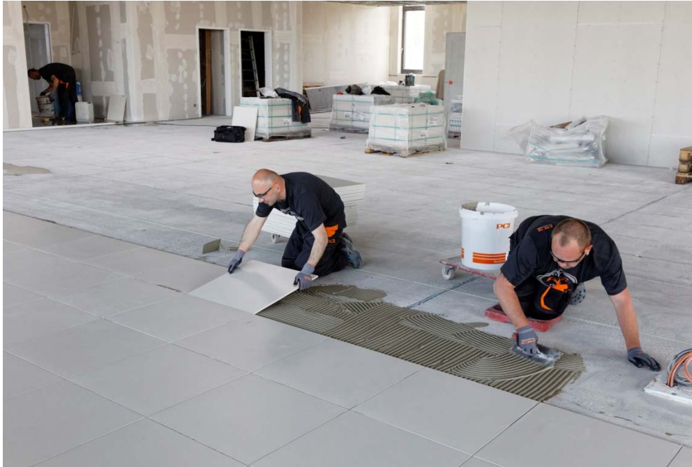
Fig. 5: After the adhesive has been applied, the tiles are positioned in the adhesive bed with a slight pushing motion and aligned.
