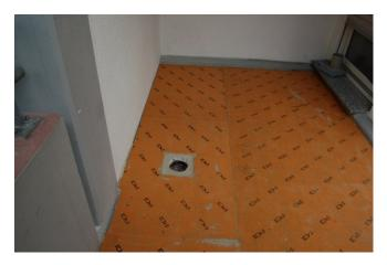
PCI Pecilastic U membranes were used for waterproofing. The entire surface of the membranes was bonded using PCI Nanoflott light adhesive. PCI Pecitape and PCI Seccoral 1K were applied to the joints between the individual membranes.
