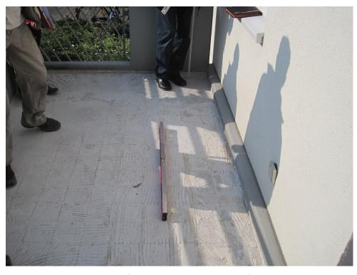
Following the removal of the old tiling, a slope of about 1% was created and the surface was primed using PCI Gisogrund Rapid.
