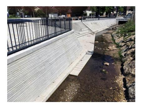
For the layered granite masonry the craftsmen used PCI Pavifix CEM ROC cementitious paving mortar for both setting and pointing.
