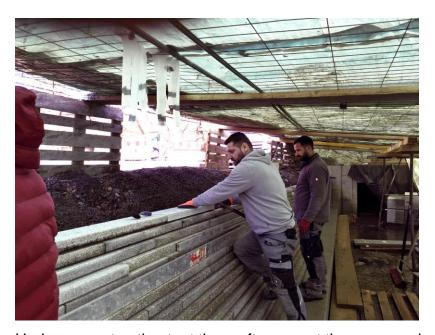
Under a construction tent the craftsmen set the masonry in winter temperatures. The special challenge was posed by the particularly narrow joints of just five millimeters. With the crack-free hardening mortar PCI Pavifix CEM ROC the joints could be executed reliably and without breaking out.
