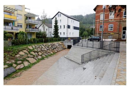
In winter 2019, the construction company Hoyer from Kirchheim unter Teck carried out the construction work with building materials from PCI: Granite slabs on approximately 60 square meters and a layer masonry on circa 80 square meters were laid.
