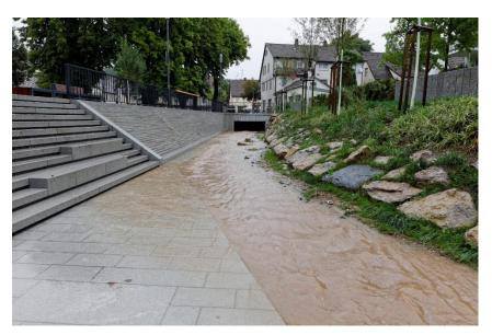
The grey natural stone facing at the Götzenbach crossing was laid with PCI Carrament and grouted with PCI Pavifix CEM ROC.
