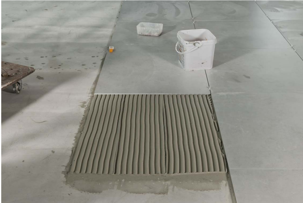
Fig. 2: The flexibility of the tile adhesive allows it to absorb stresses caused by the substrate and by temperature fluctuations.
