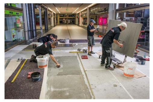
PCI Flexmörtel S2 Rapid, the tile adhesive used by the CERA-XXL team, reliably compensates for stress from the substrate and allows the new tiling to be walked on after only five hours thanks to its short setting time.
