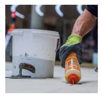
Hollows were repaired and joint gaps were filled with odourless PCI Apogel SH silicate casting resin.
