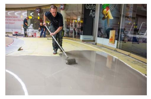
Level markers were positioned before levelling the substrate. The craftsmen then poured the PCI levelling compound onto the substrate and distributed the compound evenly over the prepared area.
