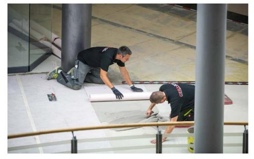
In order to compensate for later stress and cracking of the substrate, the craftsmen laid PCI Pecilastic isolating underlay on the thoroughly prepared substrate using highly elastic PCI Flexmörtel S2 Rapid adhesive.
