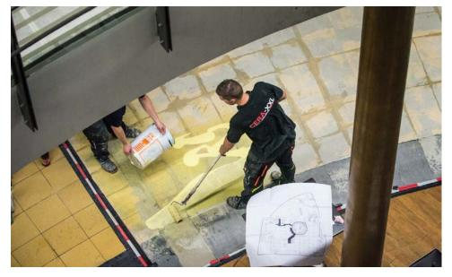
The primer used was PCI Gisogrund 303. This extremely low-emission solvent-free special primer can be applied easily by rolling or brushing. Thanks to its bright signal colour, it is easy to recognize.
