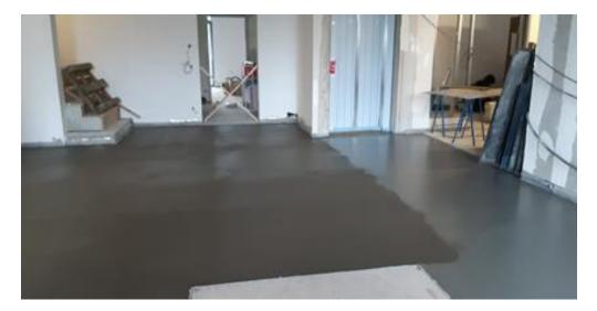
Image 3: The prerequisite for perfect execution for large formats is an absolutely even surface. Initially, PCI Gisogrund and the special filler PCI Periplan Extra were used. The surface was then filled with PCI Seccoral 2K Rapid.
