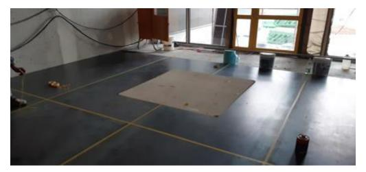
Photo 4 + 5: The steel slabs were laid with PCI Flexmörtel S2. The highly flexible mortar compensates for temperature fluctuations and substrate tension and has a very high adhesive tensile strength. For optimal adhesion of the tile adhesive to the back of the steel slab, it was primed with PCI Epoxigrund 390 and freshly sprinkled with quartz sand. The grouting was elastic with PCI Silcoferm S.
