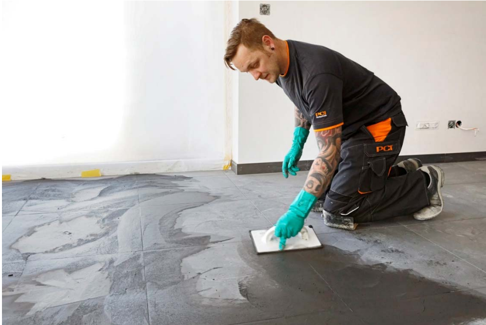
Fig. 7: The tiles were grouted using PCI Nanofug Premium. This multi-use flexible joint grout with a working time of about 40 minutes is very convenient to use and sets fast without hardening on the tile surface.
