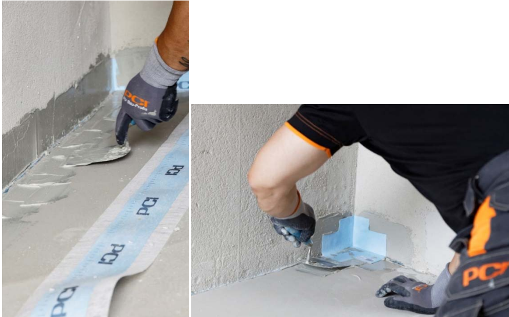
Fig. 3 and 4: Corner and connection joints, inside and outside corners as well as pipe entries and floor drains were waterproofed using PCI Pecitape waterproofing tapes, collars and corner fittings.
