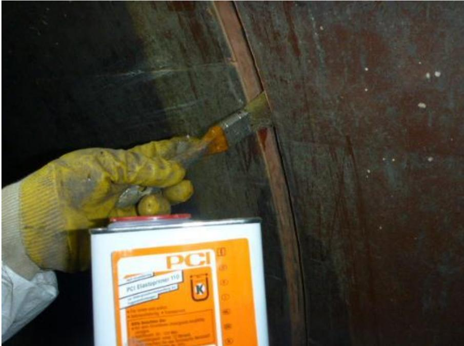
■ For a reliable 2-flank adhesion, the adhesive primer PCI Elastoprimer 110 was applied to the inner edges of the joint and the PE backing material DIN Polyband was pressed into place. PCI Escutan<sup>®</sup> TF was used as a polyurethane sealant to re-seal the 84 socket joints.
