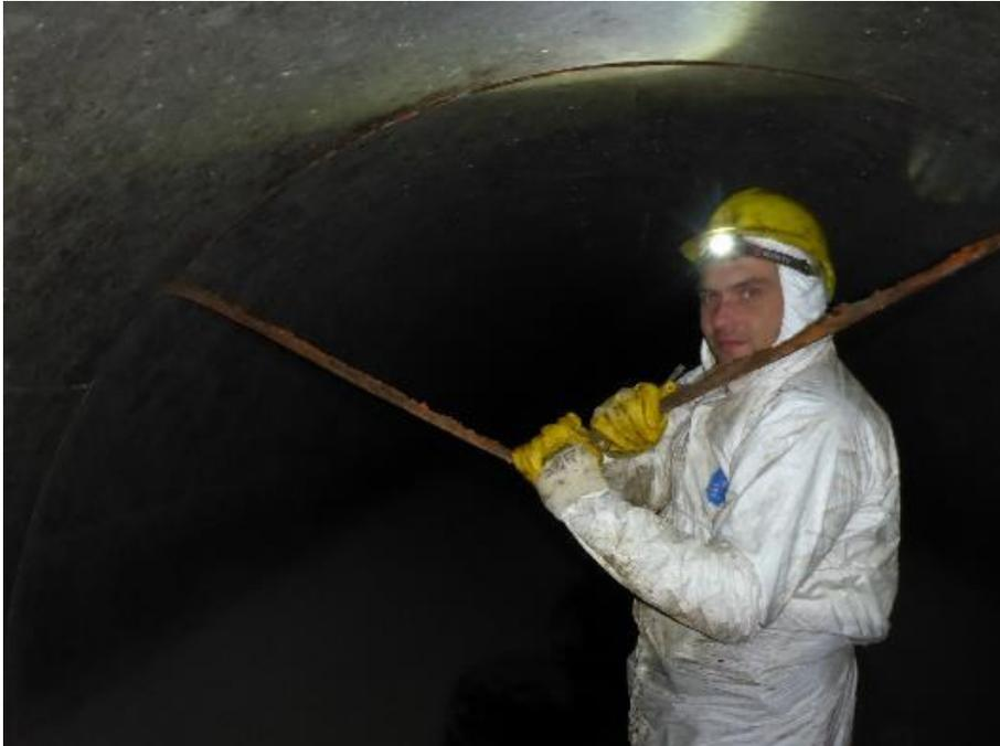
After the canal was closed, the craftsmen removed the old joints. ([Link to high resolution Photo](#))
