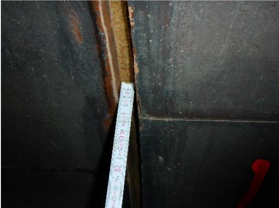
The joints were dismantled and cleaned, the joint depth was measured.
