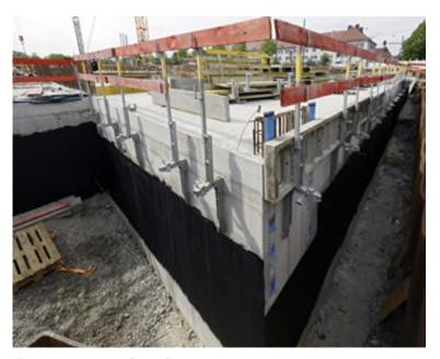
For the waterproofing of the underground parking garage, the contractor Lindermayr GmbH & Co.KG called in PCI Augsburg GmbH. Three PCI advisers provided support during the planning and construction phases.
