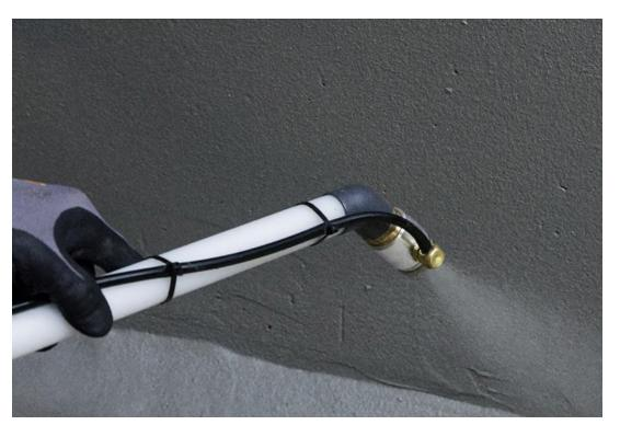
The contractor used PCI Barraseal Turbo for waterproofing the interior walls. This reactive waterproofing product has very good adhesion, sets fast and can be sprayed on quickly and easily.
