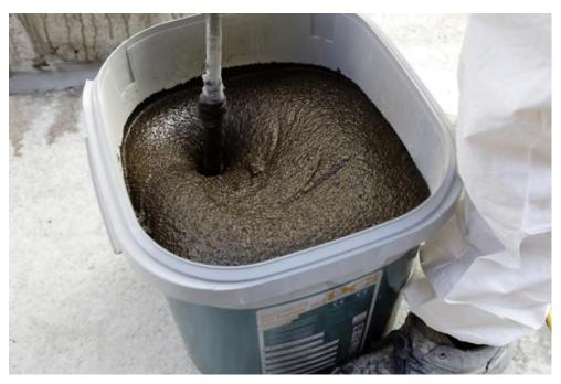
PCI Pecimor 2K can easily be mixed to form a homogeneous mass using the PCI anchor stirrer and can be applied effortlessly.
