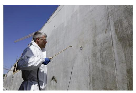
The substrate was prepared by applying PCI Pecimor Betongrund special primer.
