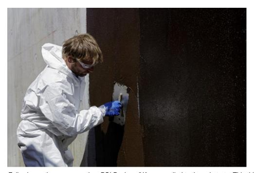
Following optimum preparation, PCI Pecimor 2K was applied to the substrate. This thick bituminous coating product meets the requirements of DIN 18533-3 and is tested in accordance with EN 15814 as well as the test requirements for the general approval of the construction authorities for products used for waterproofing structures at the transition to building elements made from concrete with high water penetration resistance.
