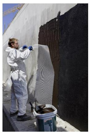
Two coats of PCI Pecimor 2K are always applied – by trowel or spray. PCI Gewebebahn fabric is inserted in the freshly applied first coat with a 10 cm overlap. The second coat is applied after the first coat has hardened.
