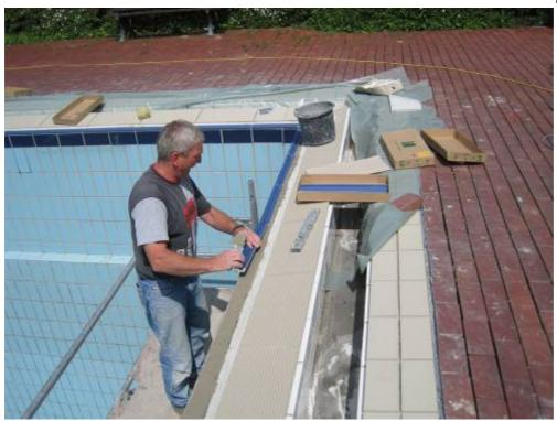
Egon Pfuhl, skilled employee and tile laying professional of the Hoffelner company, is cementing blue System Finland II stoneware handhold-pieces by manufacturer Agrob Bruchtal, a Deutsche Steinzeug company. The corresponding grooved edges are also a part of the System. Visible on the far side of the channel: Chroma NonSlip tiles 25/12.5 (colour 69 oatmeal) with slip resistance -/B.
