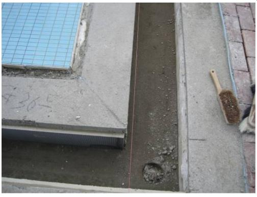
An approach that has already proven itself in scores of restoration projects – in the swimming pool sector too: levelling mortar with PCI Novoment Z1 fast setting cement plus aggregate grain in the overflow channel as well as in the pool's raised edge section and in the pool surrounds.
