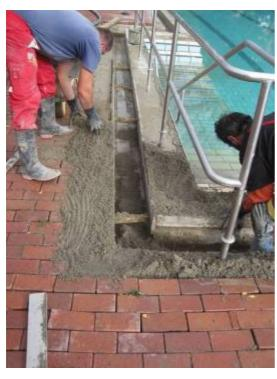
Due to the swimming pool's fixed seasonal opening dates time was pressing. This is why fast setting screed cement PCI Novoment Z1 plus aggregate grain is needed for the mortar that tile company Hoffelner's employees are laying here. Advantage: The reliable professional fast setting cement stays workable for a long time and then sets quickly. PCI Novoment Z1 can be overlaid with ceramic coatings as early as after approx. one day.
