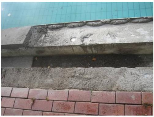
Substrate before levelling with PCI Novoment Z1 plus aggregate grain. The substrate had to be prepared "with maximum grip"; PCI Repahaft was used as the bonding agent for the levelling mortar.
