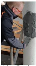
The freshly applied reprofiling with PCI Nanocret R4 Rapid meets all the compressive and adhesive tensile strength requirements as well as safeguarding structural safety.
