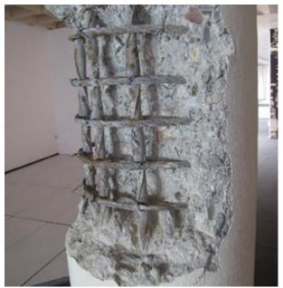
In order to ensure the structural safety of large areas with exposed reinforcement, reprofiling had to be completed very rapidly.
