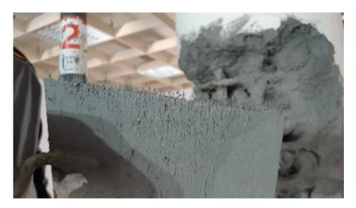
The fiber reinforcement of PCI Nanocret R4 Rapid ensures sustainable stability. The repair mortar can already be worked over after two hours.
