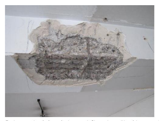
For the conversion of a former furniture store in Siegen, the condition of the structure had to be verified. For this purpose, cores were drilled in ceilings and the reinforcement of supports and beams was exposed.
