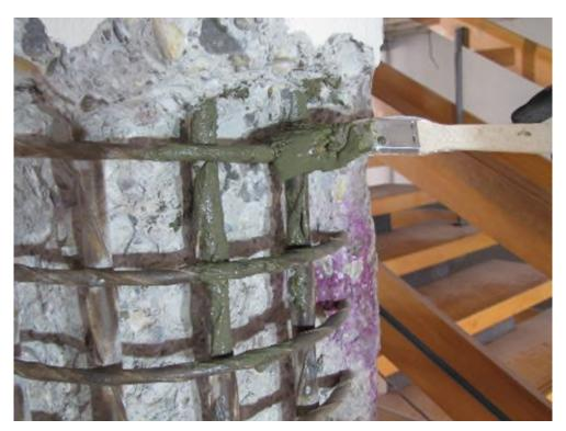
PCI Legaran RP was applied for corrosion protection. Carbonation was identified by spraying phenolphthalein indicator solution onto the structure.
