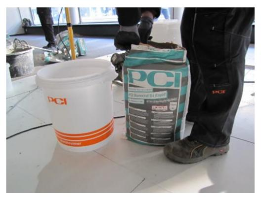
For the fast and reliable reprofiling of all the exposed areas, PCI application technician Stephan Leistner recommended the fast-setting repair mortar PCI Nanocret R4 Rapid.
