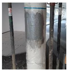
Following reprofiling with PCI Nanocret R4 Rapid, the surface was treated using foil.
